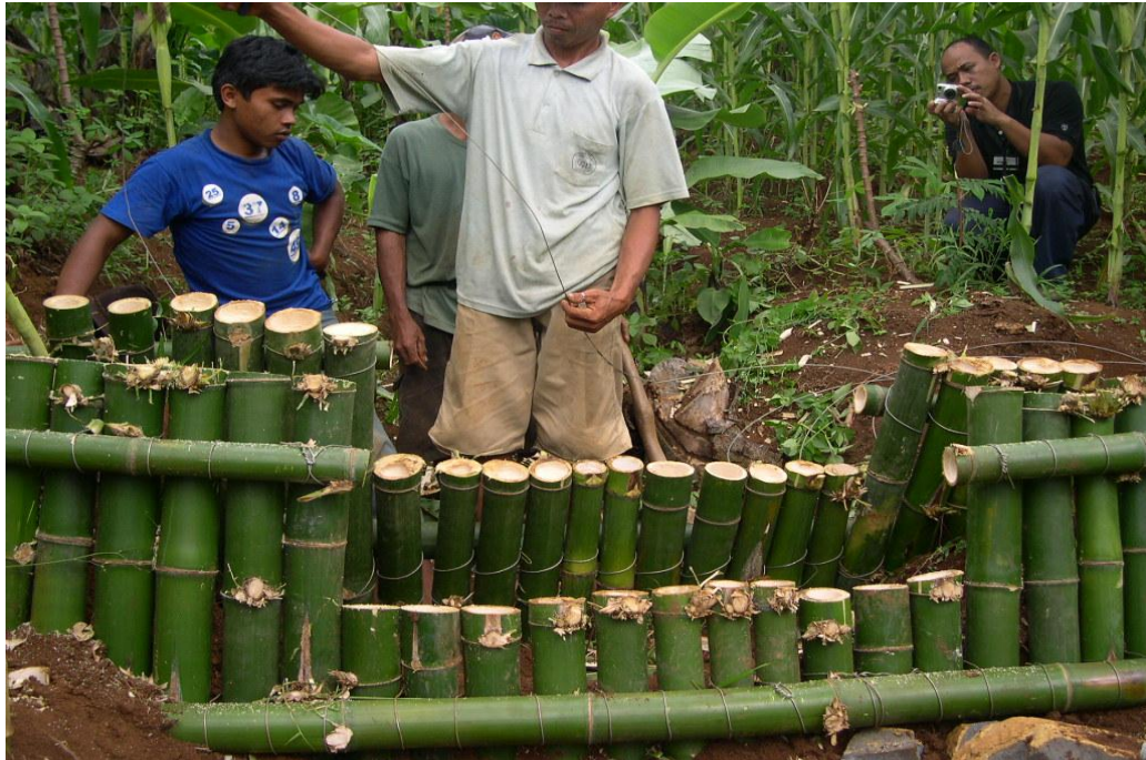
Gambar 4.45. Bio Gully Plug tampak depan di lapangan
